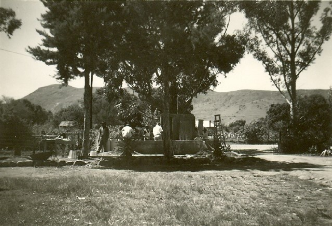
Sgt Heymans building an ablution block as they lived in tents on the “town square” – photo Col Ben Mouton.
